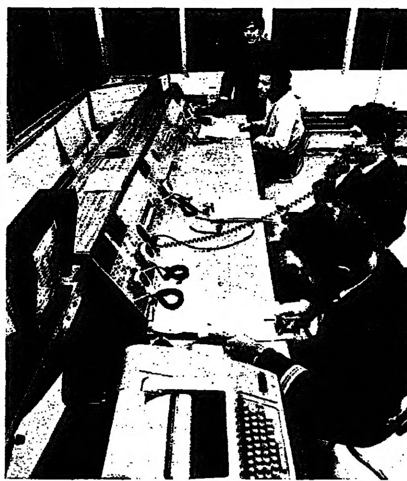
A new airport control board at Lod Airport has direct radio and other communications links with rescue services, the police, customs and all the airline companies, as well as closed circuit television surveillance of the airport. (Israel Bank)
